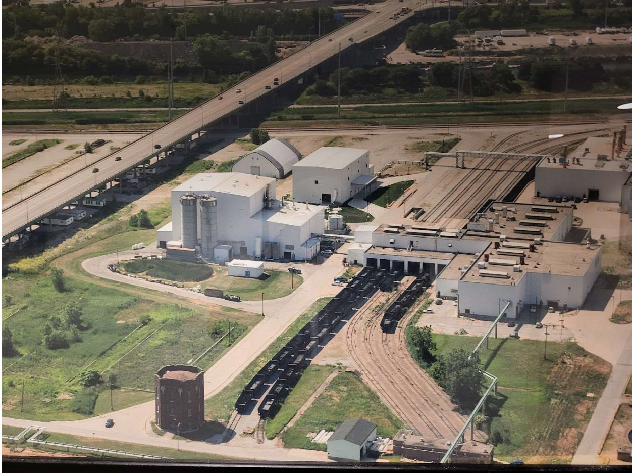
Exhibit 1. Aerial view of part of the Stickney plant looking southeasterly on June 5, 2023. At right is the centrifuge building and rail car loading facility. Left of center is the thermal drying facility. An overhead pipeline feeds centrifuge cake directly to the thermal drying facility from the centrifuge building. The Central Avenue overpass cuts diagonally, disappearing into the background. Photograph from the internet, credit Eric Jones.
