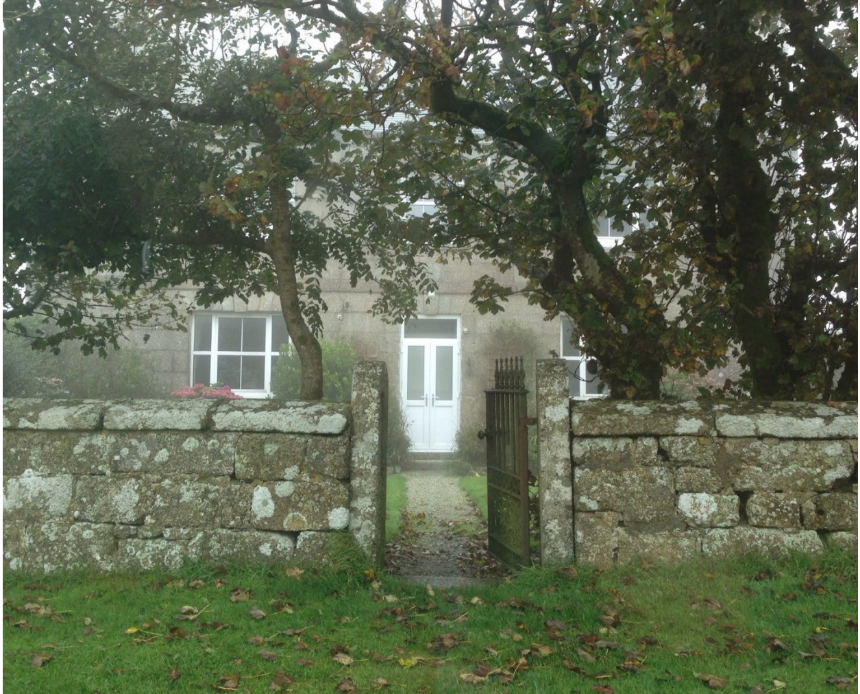
The tree offers a respite from the fog to show the gate and front entrance of the Lanyon Farm on September 23, 2013.
